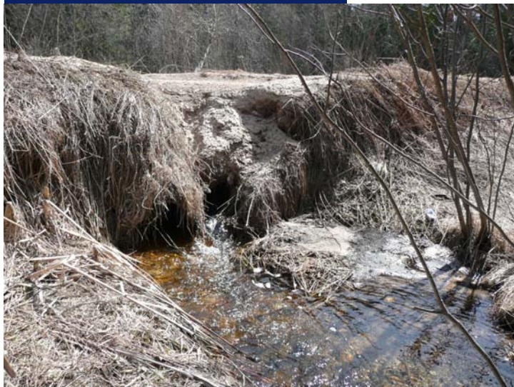
Left: The original culvert was restricting water flow and hindering fish passage. Right: Before work began, sand-laden runoff went directly into the river.
